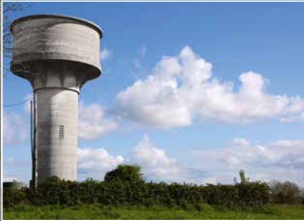
Concrete is an ideal construction material for water-industry projects (eg. facilities managing potable water)
