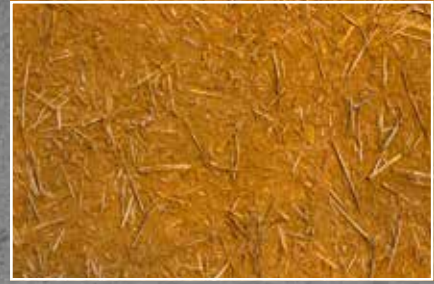
Clay wall reinforced with plant fibres.
