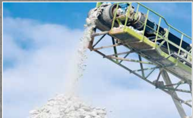
Concrete being recycled for use in road construction etc.
